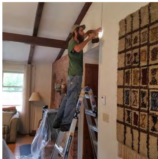
Weatherization Crew Tech, Matt Shea, seals up a client's attic
